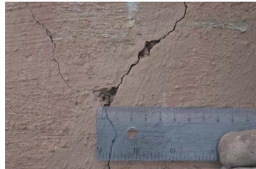
**Figure 2.** Vertical and horizontal cracks in the external wall at level + 90,00
